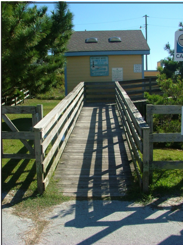
The boardwalk ramp entrance
