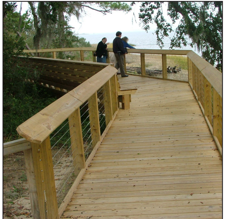
The ACCESS North Carolina program provided a boardwalk around the fort.
