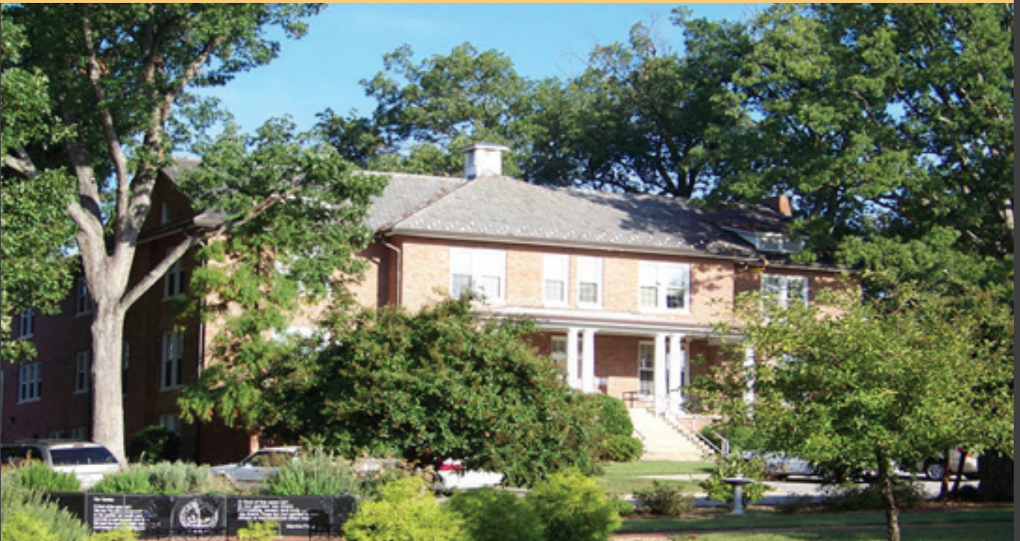
NC Division of Services for the Blind's Fisher Building and Administrative Office
